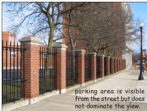
Architectural screen w/ masonry and iron fencing.
