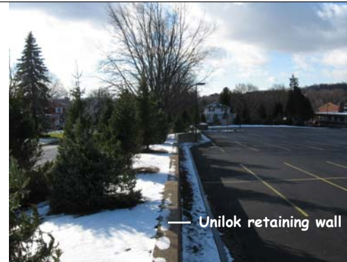
Screen system that employs an earth berm along the road (opposite residential area) and a masonry retaining wall along the parking lot. A mixed-specie planting screen is provided along top and sides.
