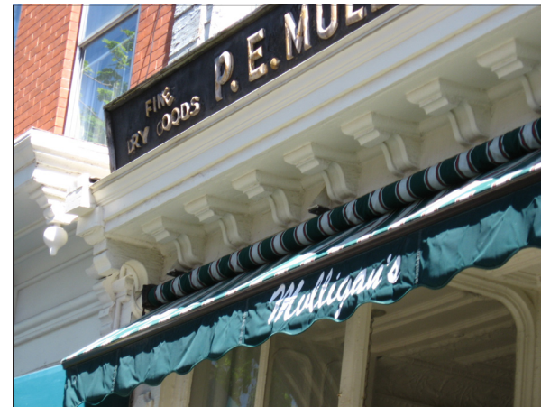
Storefront detailing with a pronounced storefront cornice, sign board above and awning nicely fitted to the storefront opening.
