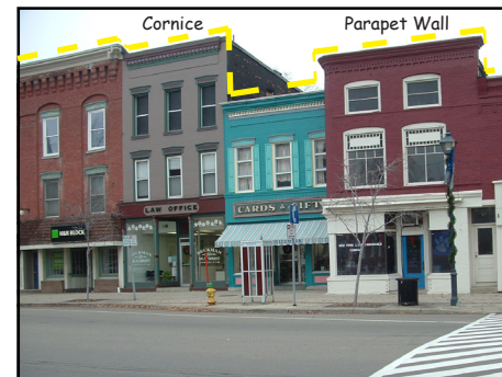
Section of Main St. in Westfield illustrating shed-type roofs with parapet or cornice elements. Note also the variable building heights.
